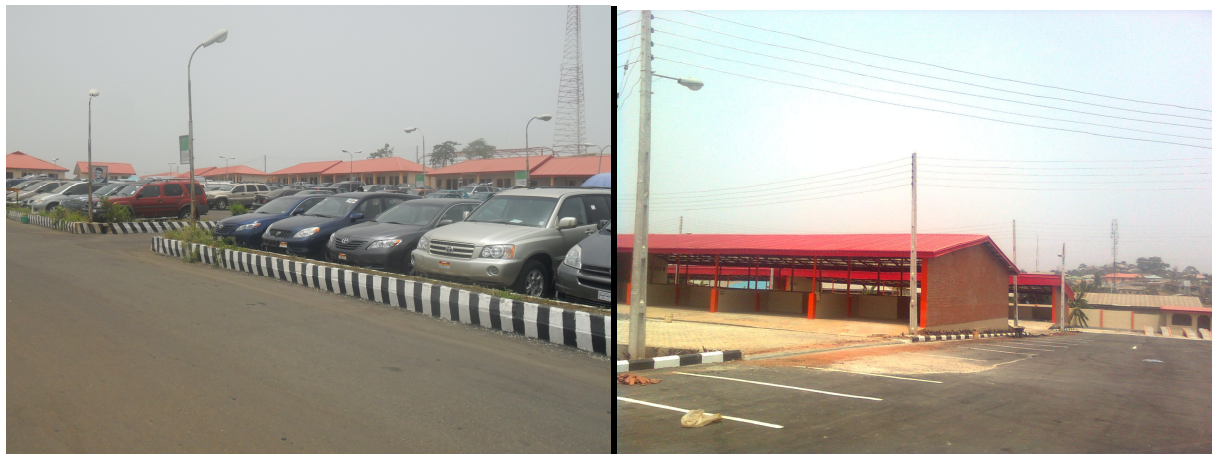
Plate 3: The Newly constructed Automart (L) and the new Mechanic Village (R) with adequate setback and air space
