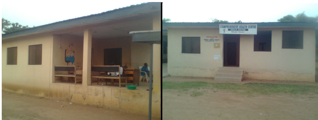
Plate 2: The Upgraded Maternity Center in Akure South Local Govt. (L) and Upgraded Comprehensive Health Center in Isolo (R)
