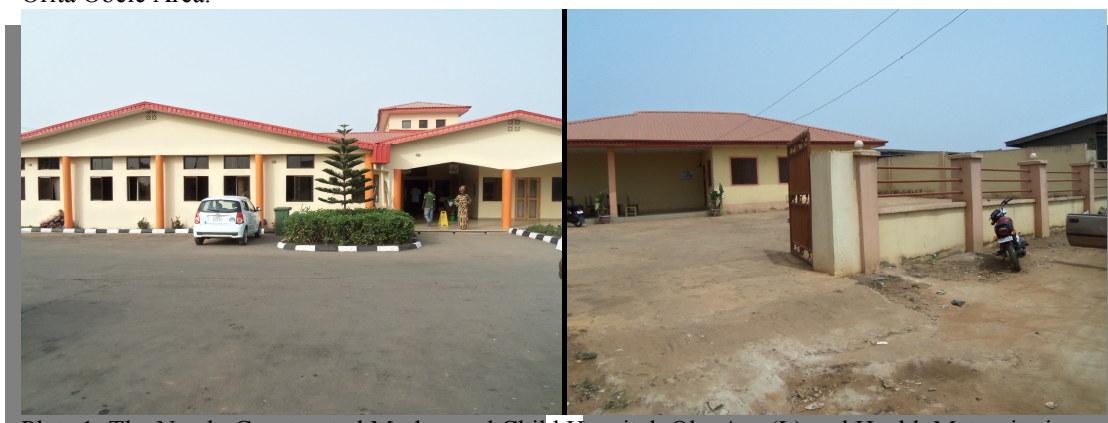
Plate 1: The Newly Constructed Mother and Child Hospital, Oke Aro (L) and Health Maternity in Orita Obele
