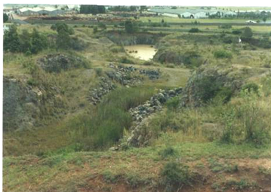
Plate 3: A dangerous pool of water collected on an unrehabilitated quarry near Raiply wood processing plant
