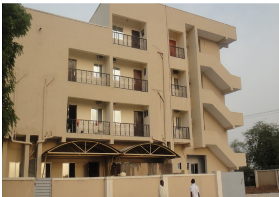
Plate 3: Sliding windows in Seven Sisters Hotel Source: Field Survey 2014
