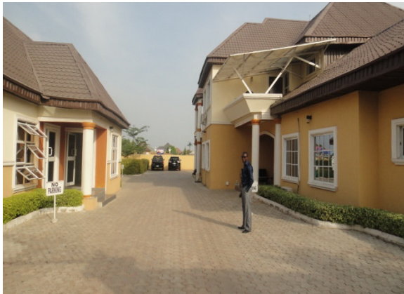
Plate1: Sliding windows in Yukuben Hotels Source: Field Survey 2014
