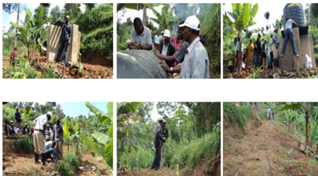
Fig 5-1: Protocol for installation of drip irrigation system the case of Kwamboa
