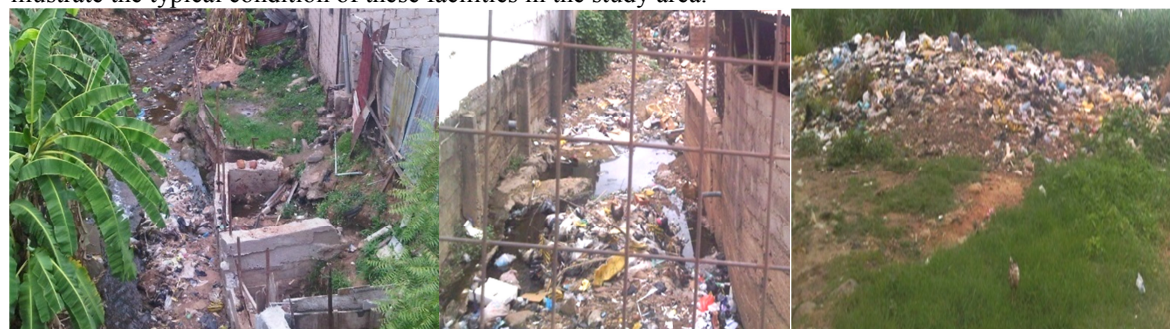
Plates 2: Condition of Drainage Facilities and Poor Disposal Method of Solid Waste in the Area
