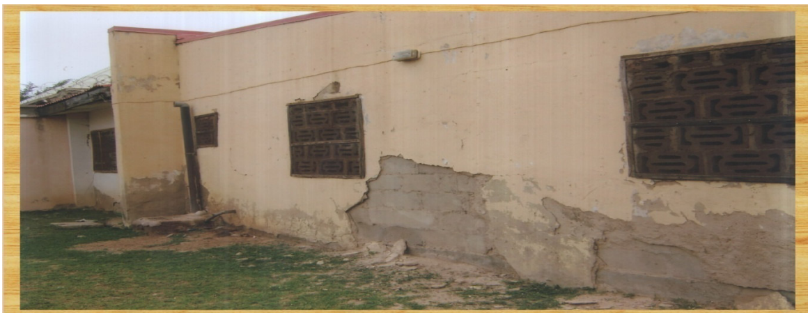
Plate 7: Picture showing part of a poorly maintained building in Igala Housing Estate Source: Authors' field survey, 2015.
