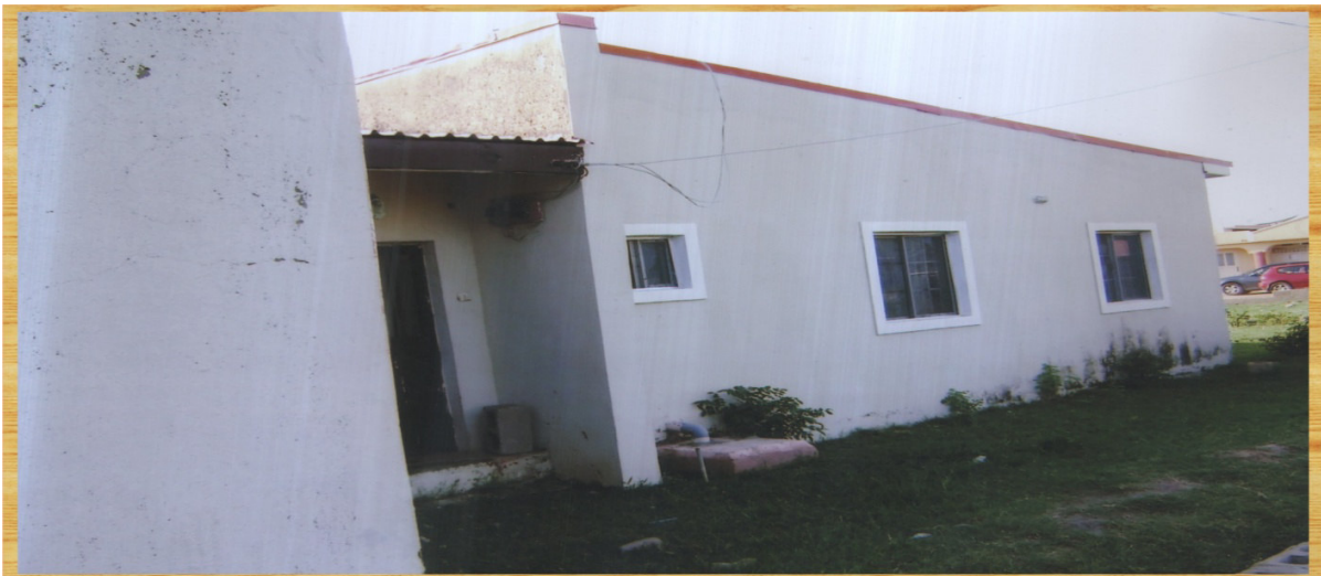
Plate 4: Picture showing part of a building in Igala Housing Estate
