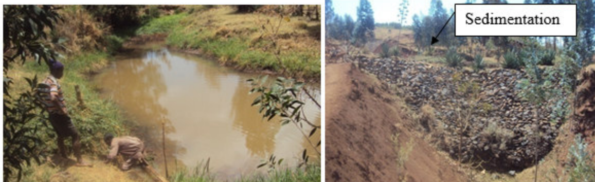
Figure 5. Farmers fetch water from SSD. Figure 6. SSD constructed on a large gully
