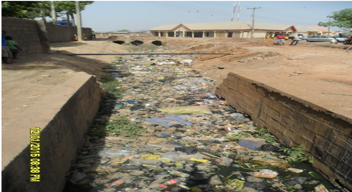
Plate 1: Blockage of Storm-water Drainage due to indiscriminate dumping of refuse in Demsawo. This is the only storm-water drainage in the area.
