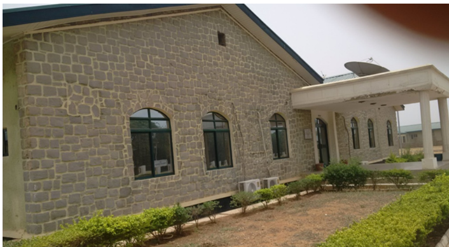
Plate iv: showing façade of faculty of medicine/ Dean's office. (Source: Authors Field work)
