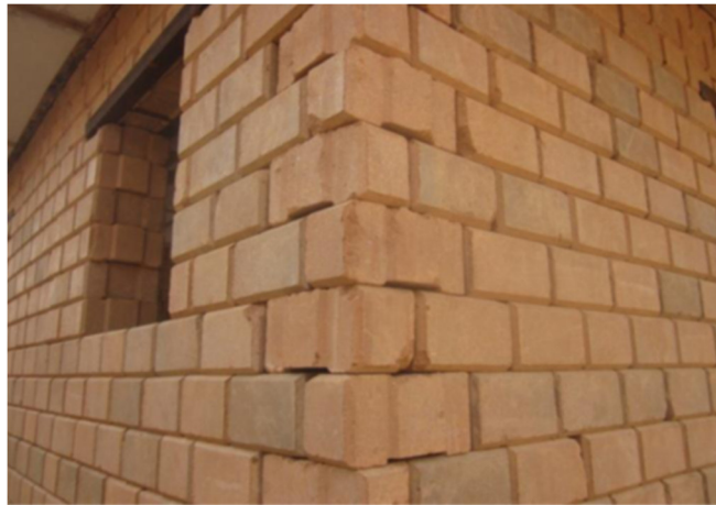
Figure 5. Dry construction using CEB
