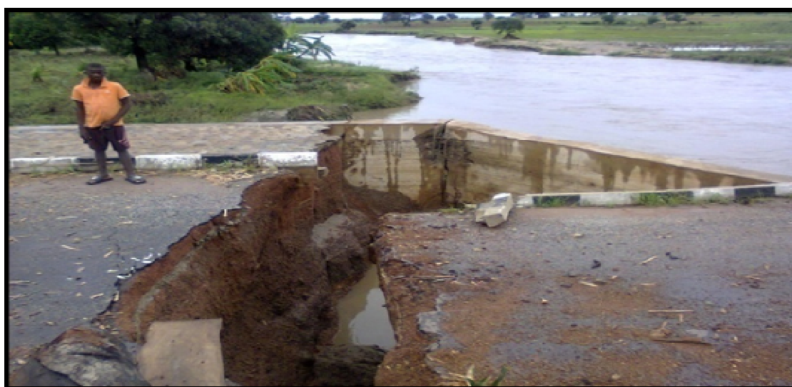
Plate 4.12 Bridge linking other Villages Source: (Buba Y. Alfred 2012)
