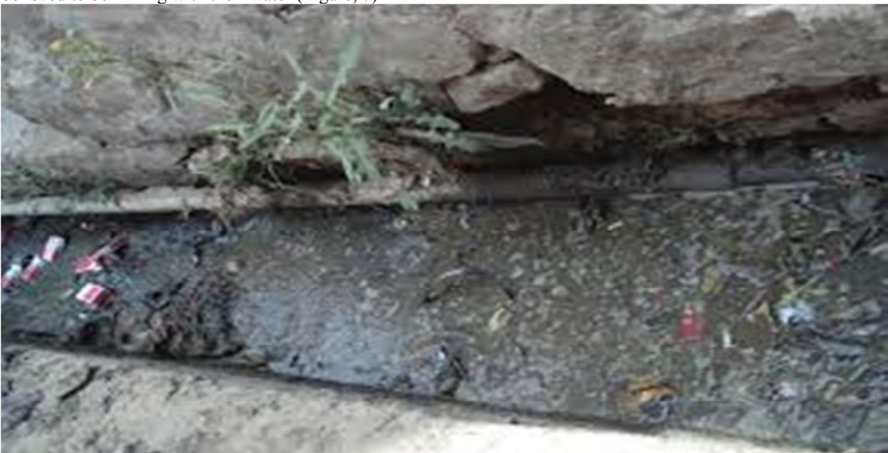
Figure 7: Drinking water pipe passes through gutter channel
