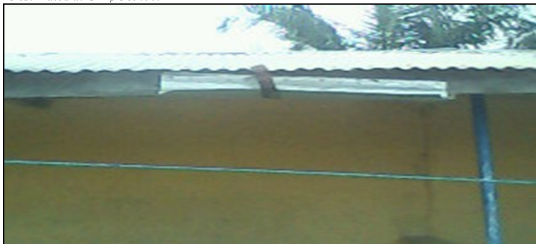
Figure 3: A Typical Rain Gutter at Fumso
