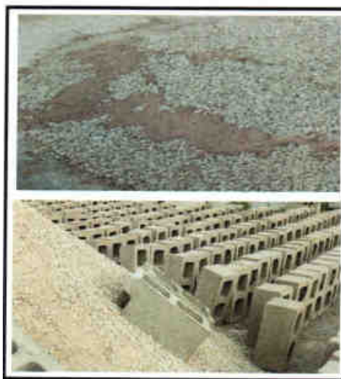
Figure 1. Composition and completion of aggregate filled stone-dust block.
