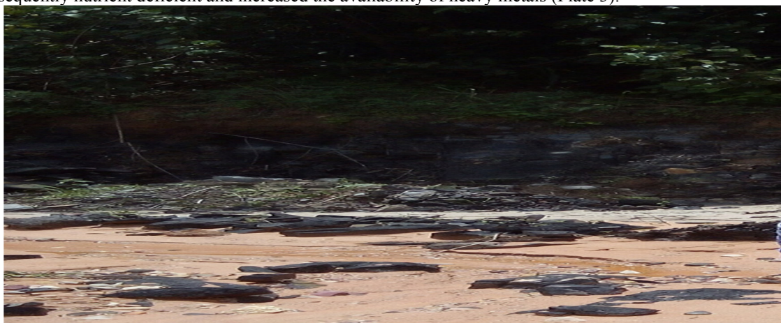
Plate 3: Evidence of Acid Mine Drainage Source: Field Study (2017)
