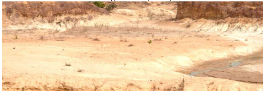
Plate1: Soil Exposed to Erosion during Site Clearing around the Mining site.
