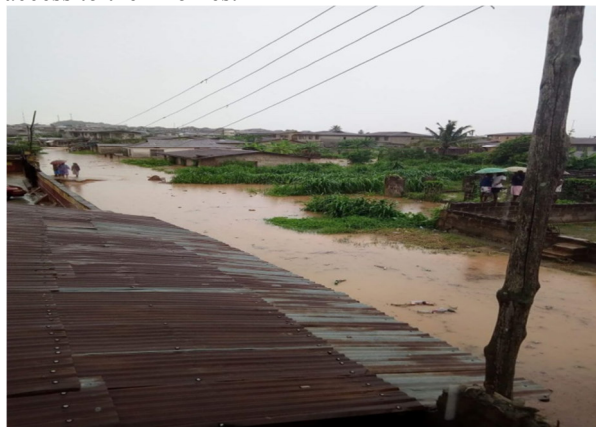
Plate 3, New Town accessing road Flooded with stagnant surface water Source, Author's archive
