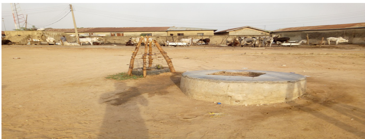
Plate2: Effluent well at Gwagwalada Abattoir, FCT-Abuja
