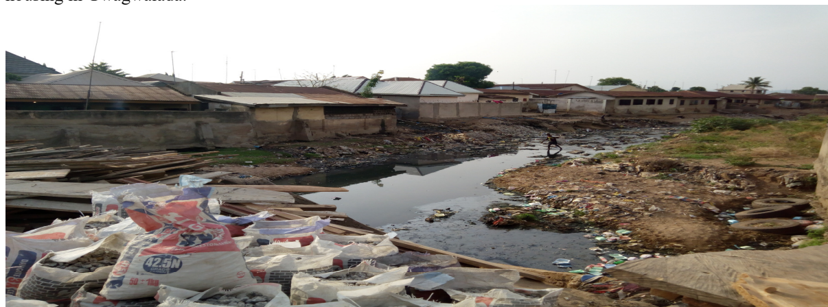
Plate 1: Un-conducive state of housing in Kutunku, Gwagwalada satellite town, Abuja-Nigeria.
