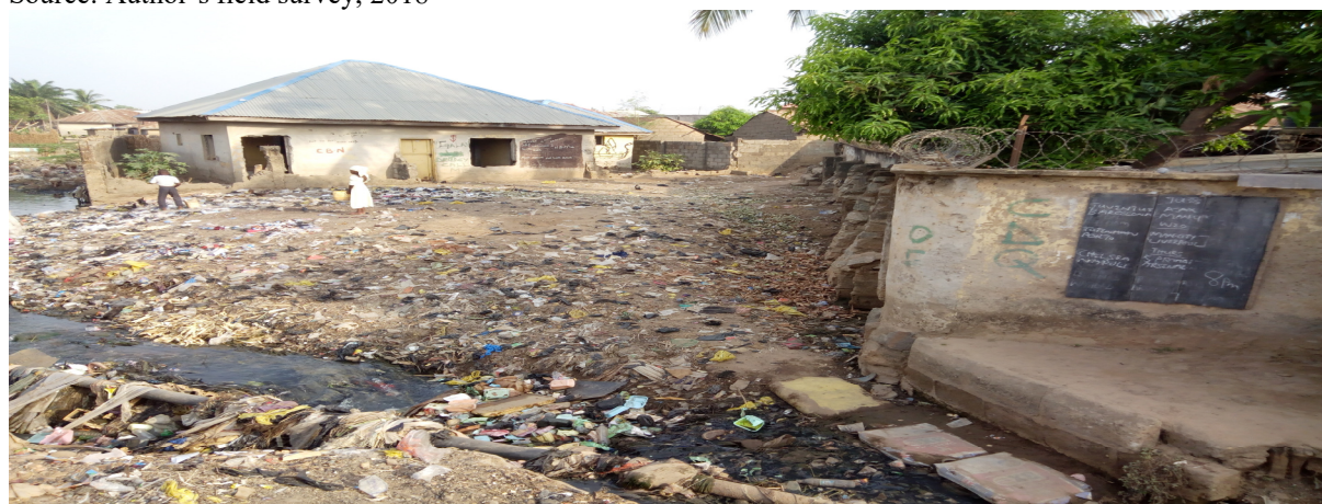
Plate 2: Poor state of housing in Angwan-Dodo, Gwagwalada satellite town, Abuja-Nigeria
