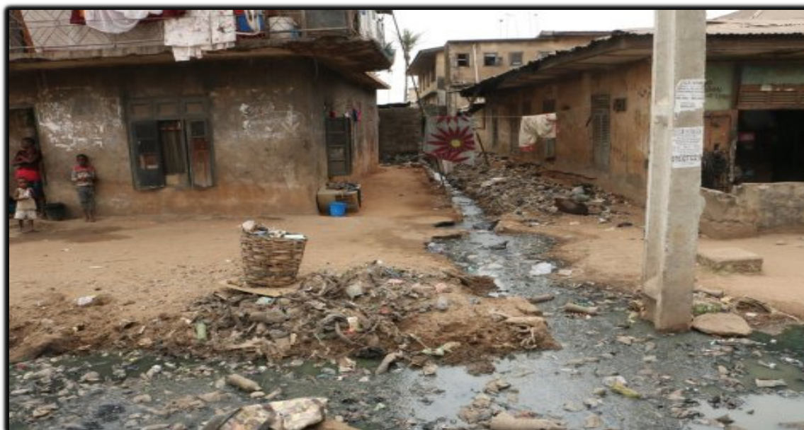
Figure 4: A cross-section of substandard residential buildings in unhygienic environment around the Olusosun dumpsite
