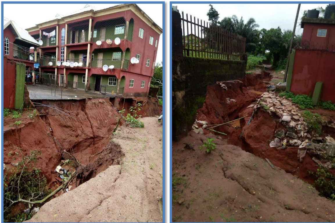
Plate 0.1: Gully Erosion Affecting the Environment in Niger Delta, Nigeria
