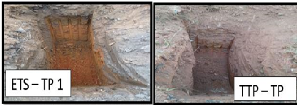
Figure 2. Typical Trial Pits in the ETS and TTP Area. Source: Authors, 2015
