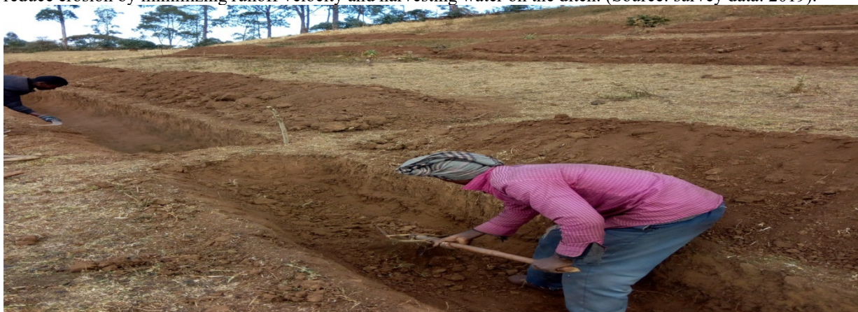
Figure 3: Fanaju bund constructed on farm lands at Tuttiti kebele
