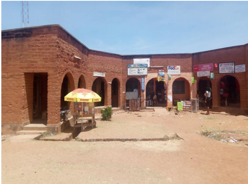
Fig 3 Exterior of building.
