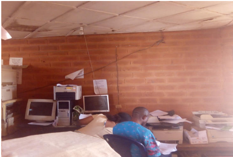
Fig 2 Interior of Building.
