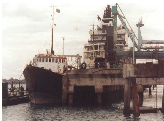
Figure 5a: Port facility
