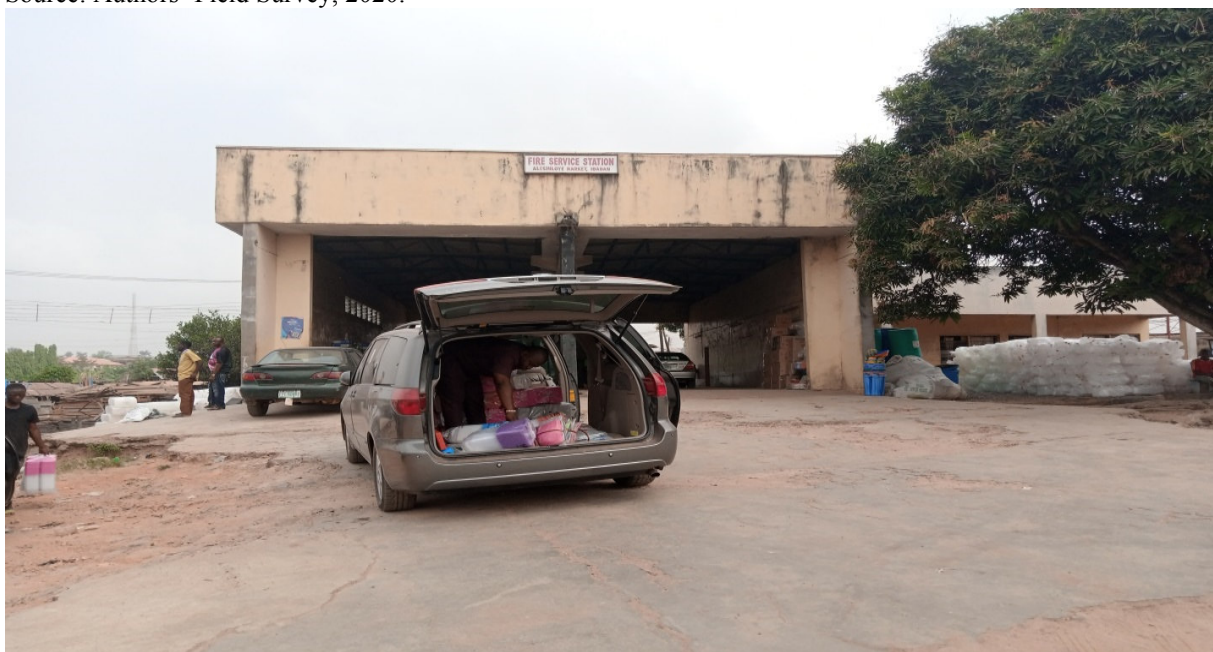
Plate 3: Fire Station in the Study Area. Source: Authors' Field Survey, 2020.
