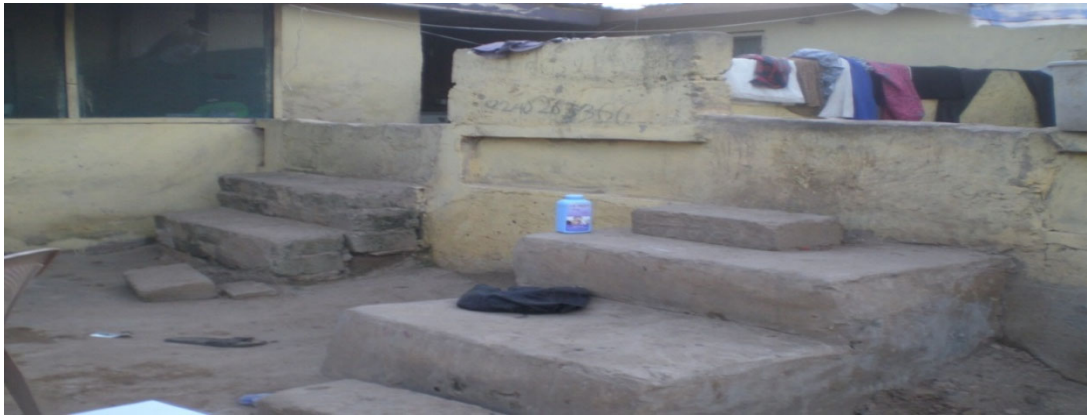
Plate 3.1: Raise Door Threshold in Awoshie to prevent flood water from room.
