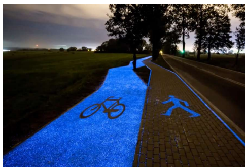
Figure 6. Concrete with photoluminescent (Olsztynska, 2017)
