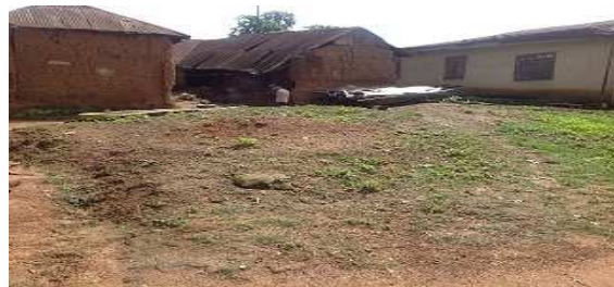
Plate 6 Laterite adobe walls used in Ilaramokin.
