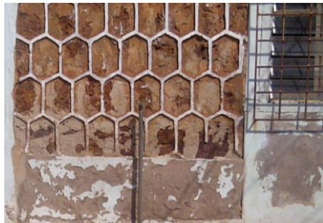
Plate 4: Traditional walling material Source: Author's fieldwork (2012)
