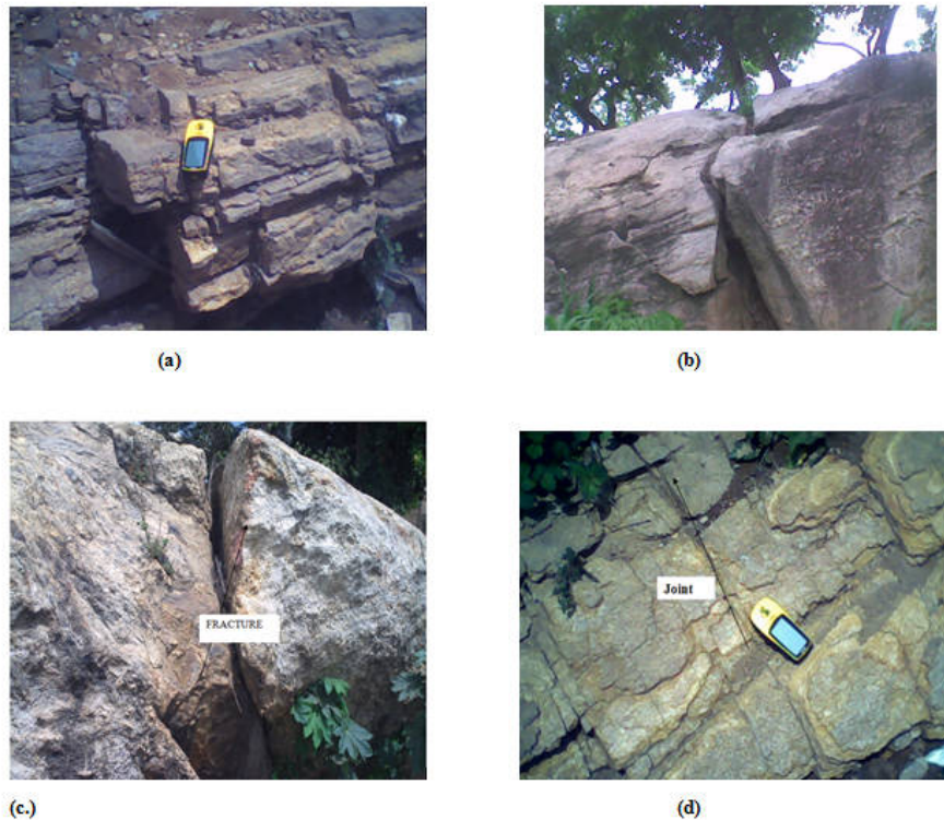
Figure 7. Lithology and some geologic structures at Oke Alapata, South-western Nigeria (a) Quartzite; (b) Migmatite gneiss; (c) Fracture; (d) Joint
