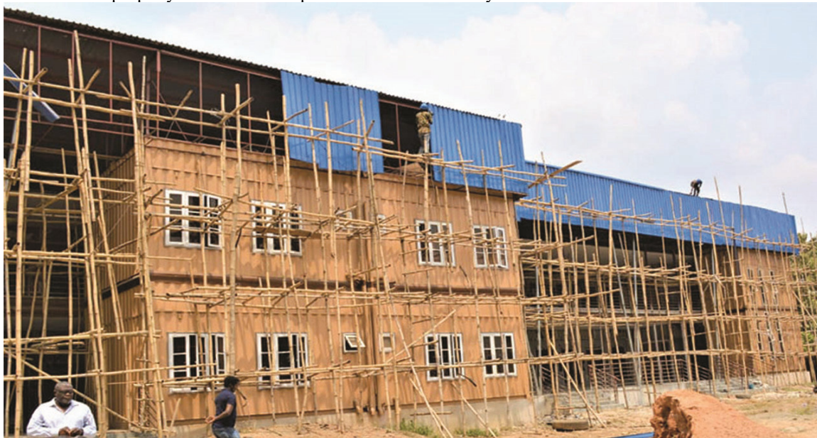
Figure 2: Ongoing Modular 12 classroom block (Nwannekanma 2022)
