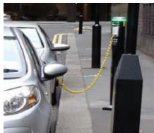
Fig. 6 On-street Electric Car Charging Station (Source: Anon., 2010)
