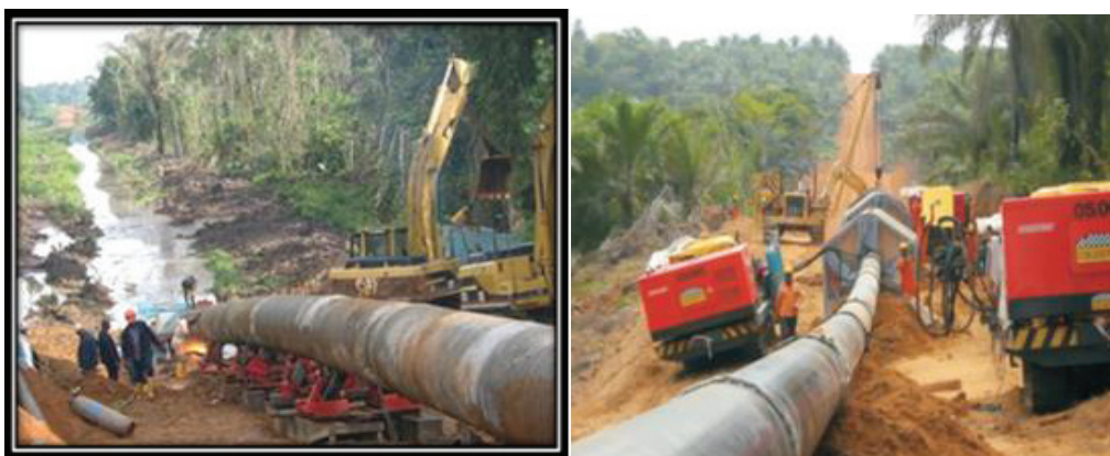
Figure 3.5: On-going Pipeline Project
