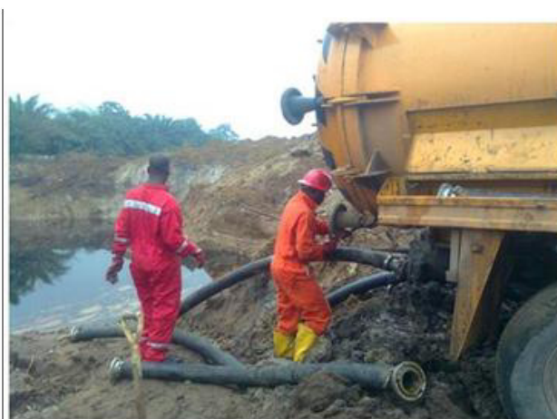
Plate 4: Free phase oil removal
