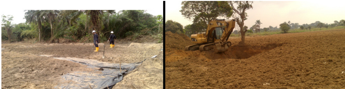
Plates 1 & 2 Land farming & Excavation in progress at one of the remediation sites in B-Dere, Ogoniland
