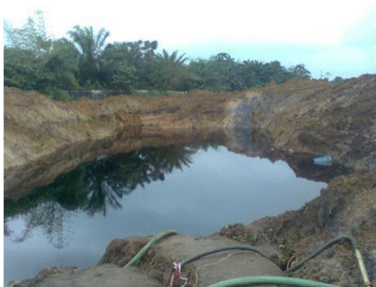
Plate 5: Deep excavated at the site.
