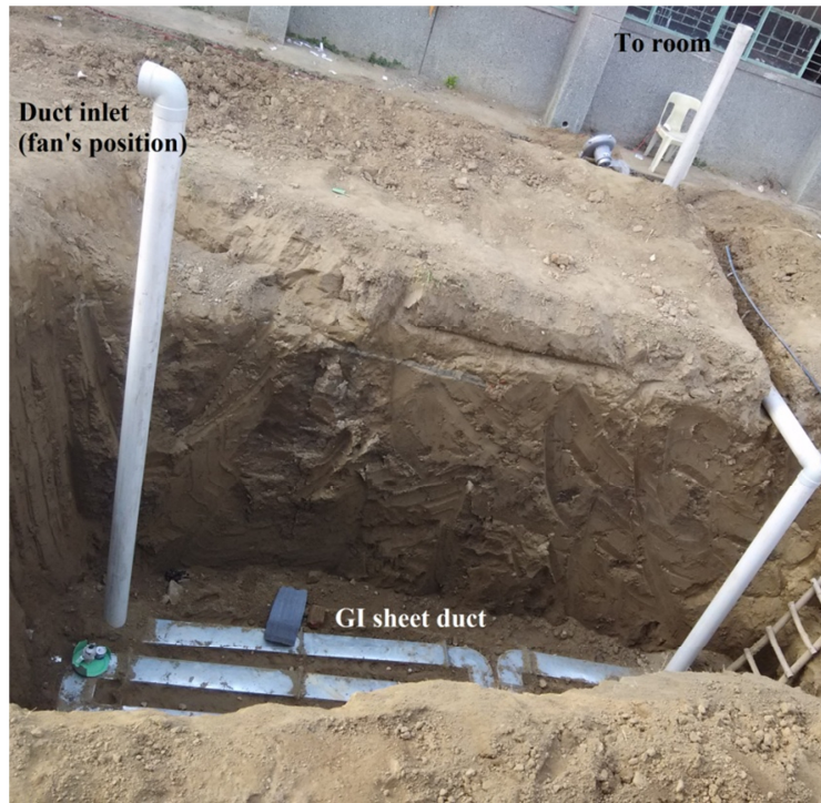
Figure 1. Prototype after being installed at the site
