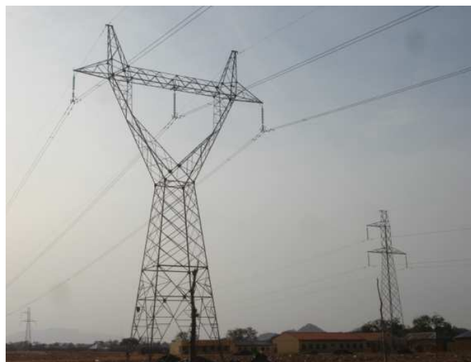
Figure 1: Jos – Gombe 330 kV (right) line and Jos – Bauchi – Gombe 132 KV (left) power transmission lines of 50-Hz which are 8m apart
