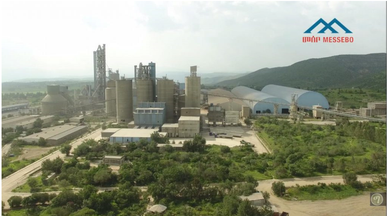
Figure 2: Messebo Cement factory
