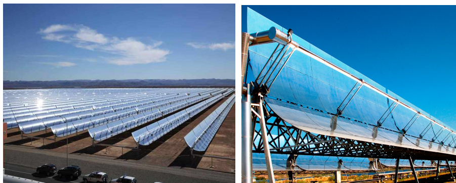
Figure 1: Concave mirrors one of system for producing electrical energy from solar radiation. Source :[3, p. 17]
