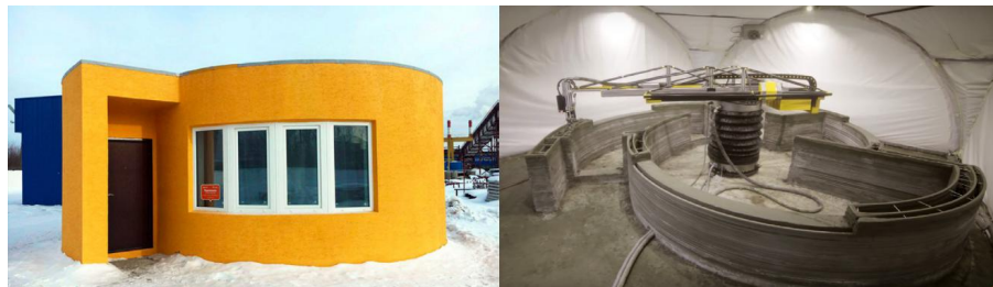
Figure 7. Figure showing a frontal view of the Apis Cor House in Russia and also showing the subsistence crafting process of Apis Cor House. Source: ( https://www.apis-cor.com/ )
