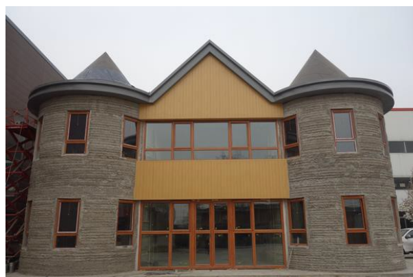
Figure 8. Two-story house entirely printed on site. Source: (Hossain et al. , 2020)
