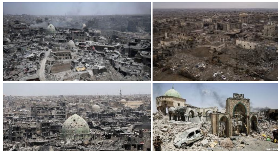
Figure .2 Destruction in the city center of Mosul. Source: (Al-Samurai and Al-Qaraghuli, 2021)
