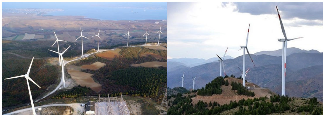
Figure 4. Views from the facility area (Kirsehir, Mucur)
