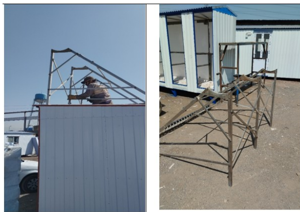
Figure 6: solar water heater installation
