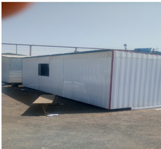
Figure 4: booths construction stages
