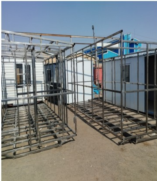
Figure 3: booths construction Structure
