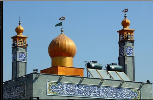
Figure 10. Polis Park's mosque, Tehran, Region 4 (Source: Tehran municipality's archive)
