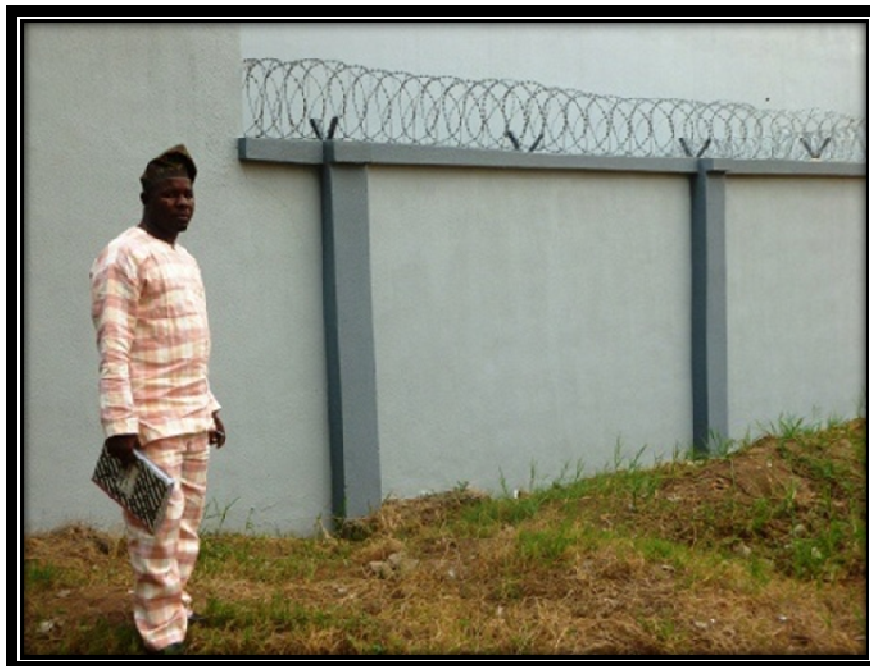
Plate 4: A Typical Fence that Dwarfs Building in Urban Areas
