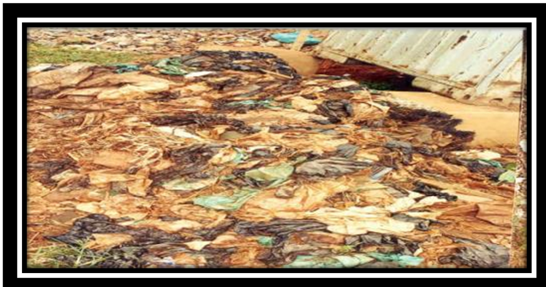
Plate 4: Blockage of drainage channel at Omagba, Onitsha Source: Anierobi (2010).
