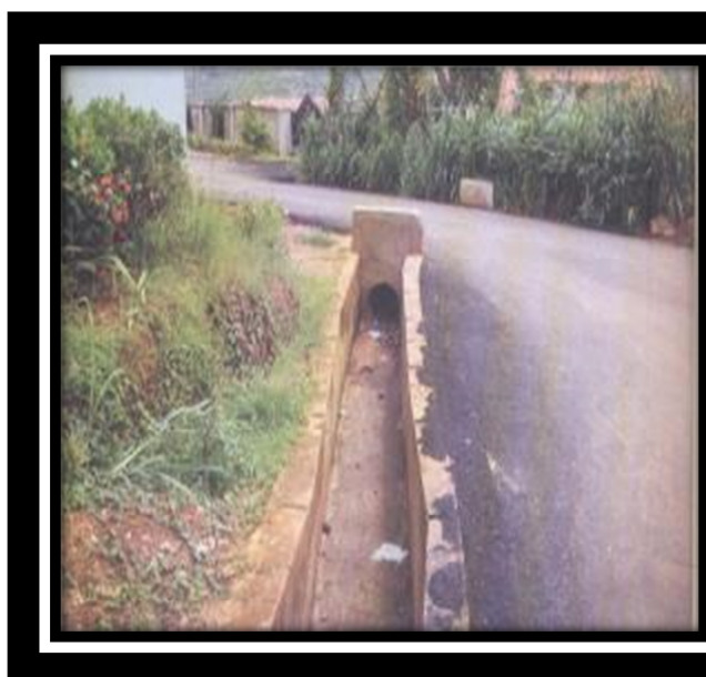
PLATE 6: Shallow and narrow Drainage Channel in the city Channel in the city Source: Anierobi (2010).
