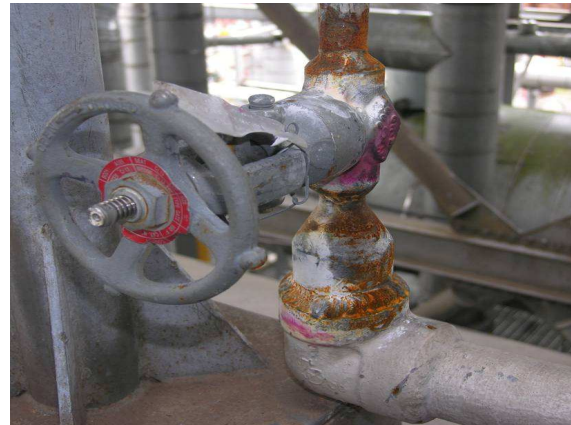
Figure 2: Repaired Reducer Nipple
