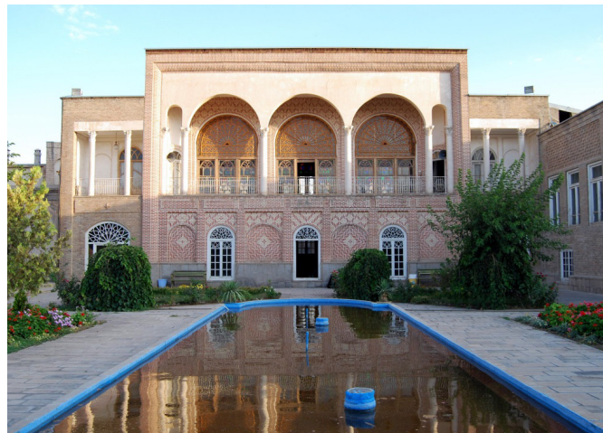
Figure 7. View of Qadaki House
