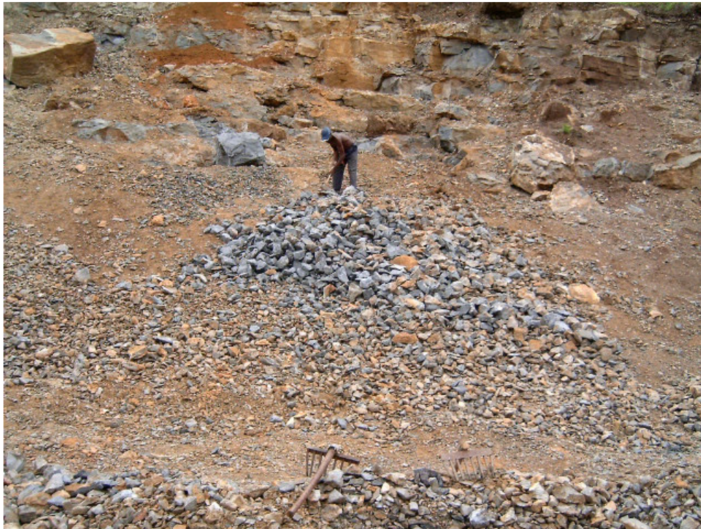
Fig. 3: The manual breaking of boulders to small sized stones
