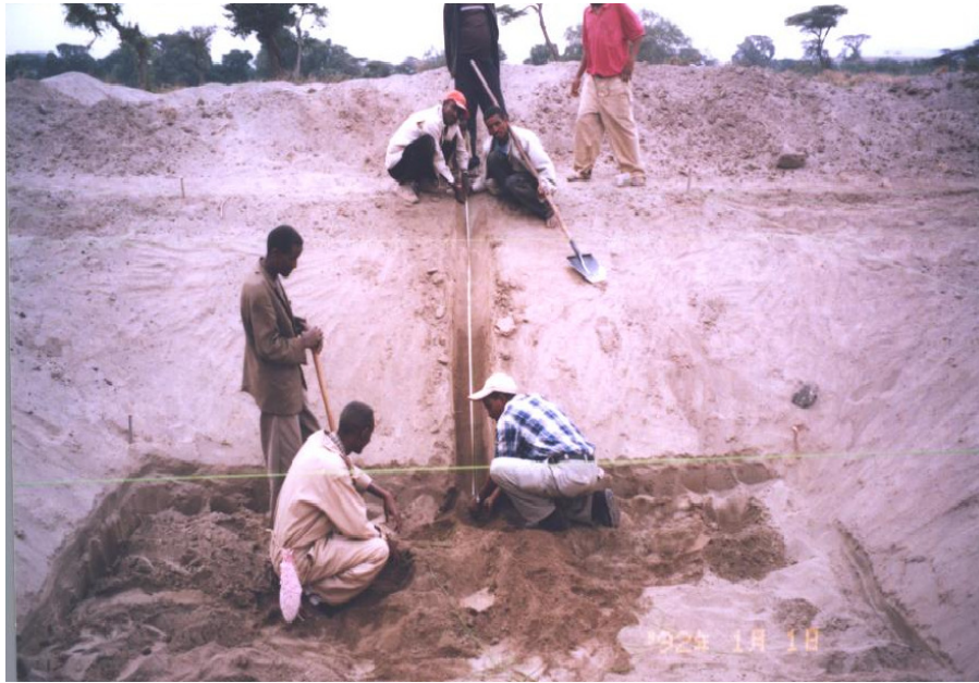
Figure 3.5 Trimming of the pond sides
