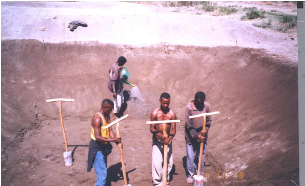
Figure 3.6 Compaction of the pond
