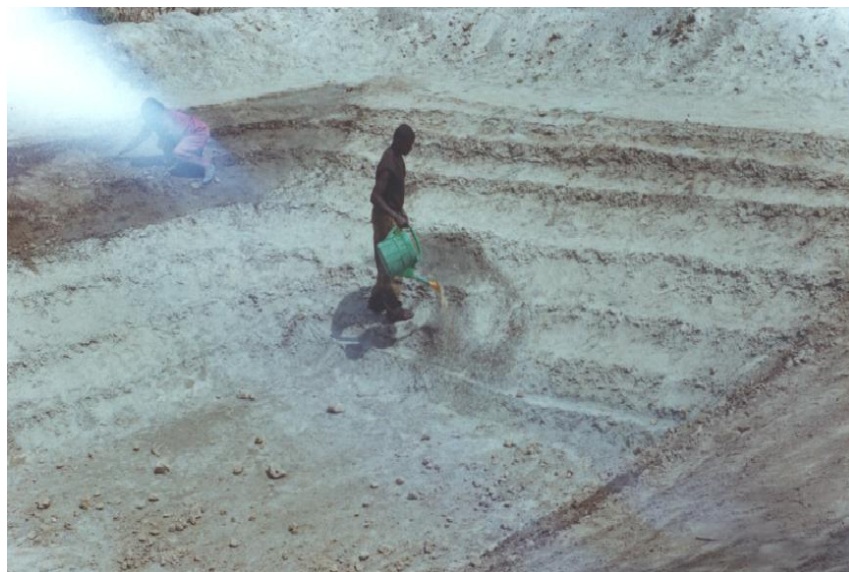
Figure 3.8.1 Preparing terraces on the pond sides
