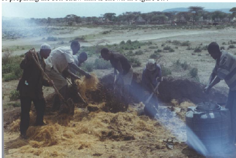
Figure 3.9 preparation of the soil-straw mix
