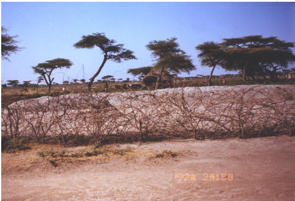
Figure 3.11 Fencing of the pond (typical of all four ponds).
