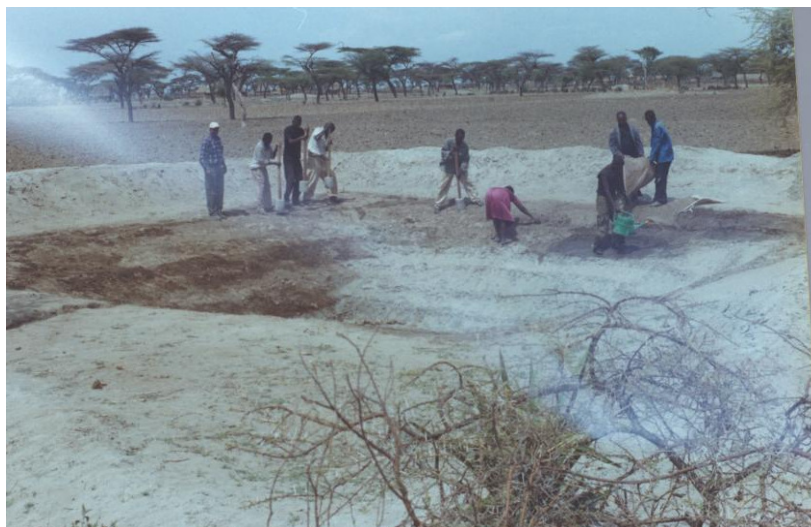
Figure 3.8.2 Treatment by termite mound and compaction
