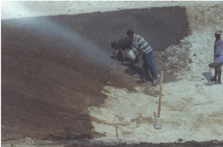
Figure 3.10 Treatment by soil-straw mixture
