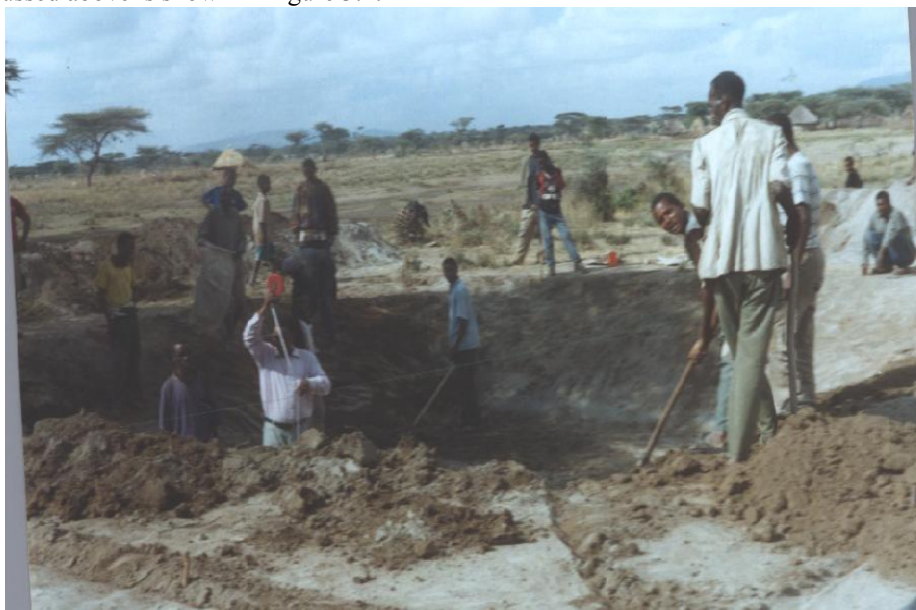
Figure 3.4: Pond excavation control
