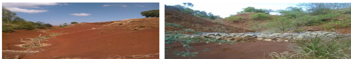
Figure 1: Gabion Structure to Conserve Soil and Water in the Study Area
