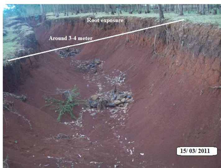
Plat 4: Active gully damage in Abay-Sangib Kebele
